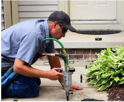
**HMI foam specifically designed for joint/slab stabilization has a very long reaction time and minimal expansion strength. It will take longer to expand, allowing for better coverage under the slab or down a void along a joint.**
