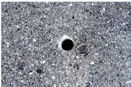
Our polyurethane foam method uses the concrete slab itself as a means of delivering poly foams that raise concrete, fill voids, and stabilize soils. A 5/8” hole is drilled through the slab into the subgrade. A tapered delivery port is installed into the 5/8” hole. The injection gun is connected to the port. The injection gun delivers the polyurethane material through the port and slab. Expansion of the material occurs within seconds, compressing loose soils and raising concrete.
